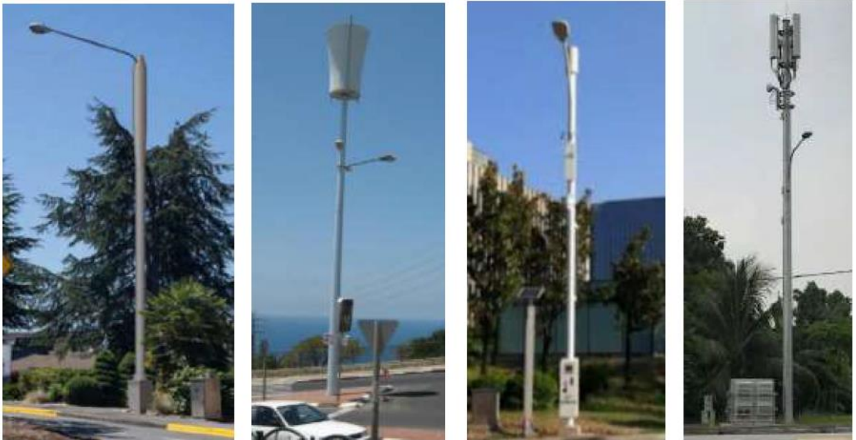
Figure 4.7 (a): Samples of new special structures; Source: edotco
